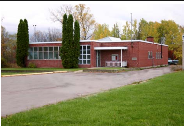
Former Canada Post Building, Batawa, ON
